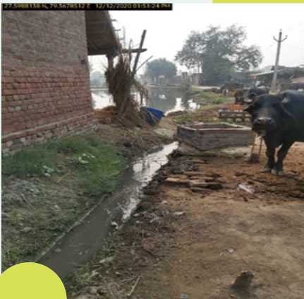
Drainage connected | UP_AKAKHEDA MOHMADIPUR_Tmp512891_027561_W1
