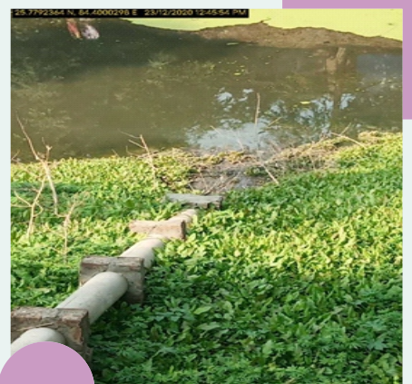
Drainage connected UP_GOPALPUR MAFL_199975_005021_W1
