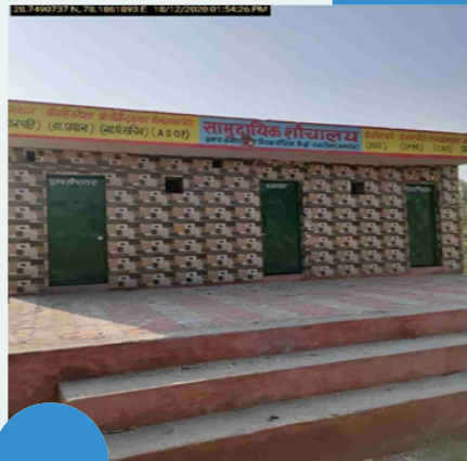
CT or PT nearby | UP_DHAURIYA AHTAMALI_Tmp512911_027771_W1
